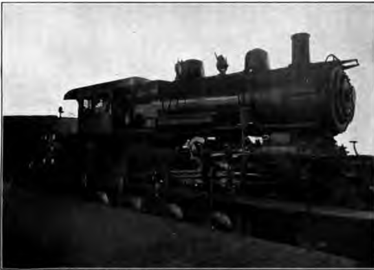
A LOCOMOTIVE UPON THE TESTING-TABLE AT THE ALTOONA SHOPS OF THE PENNSYLVANIA
